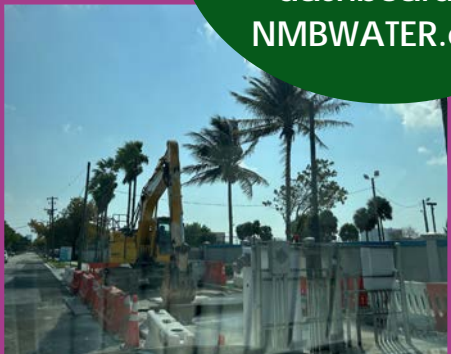
Corona del Mar Sewer System Phase 2
