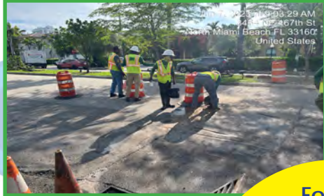
Eastern Shores Watermain Rehabilitation
