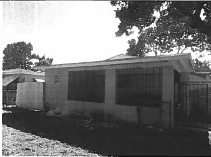
01-18-2014 HOUSE CARPORT VIEW
