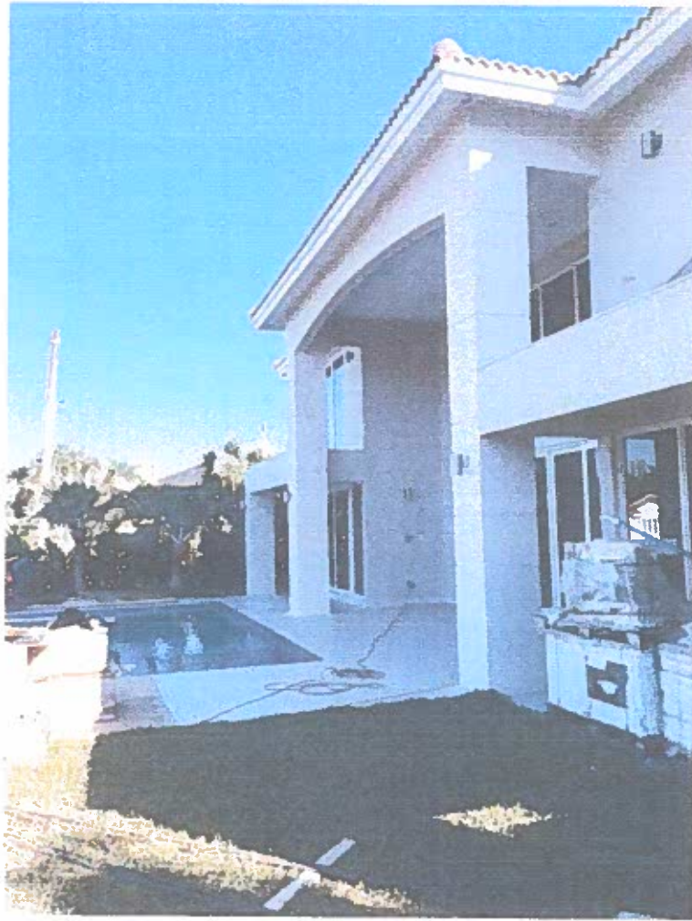
REAR VIEW DATE TAKEN 11/09/2015
