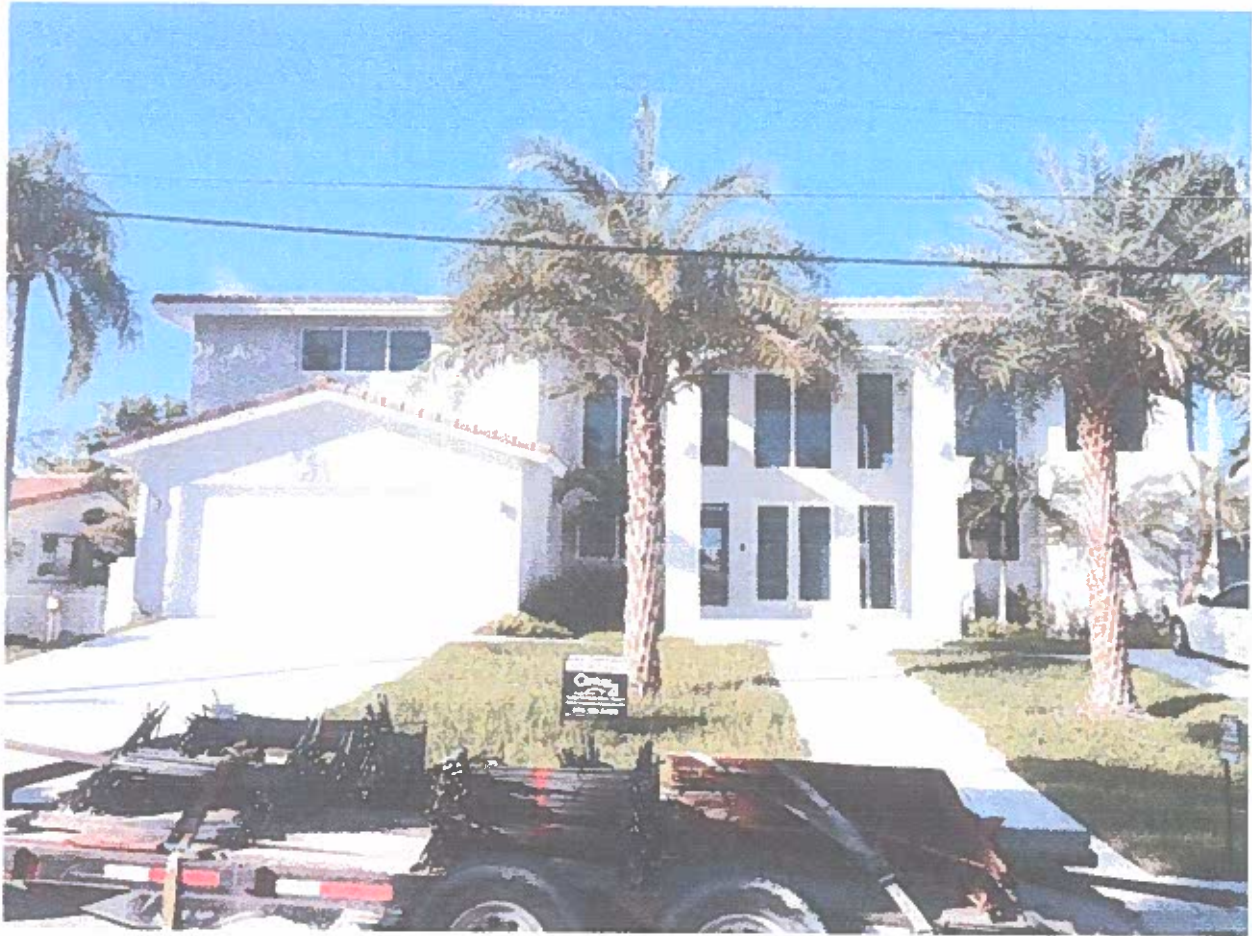
FRONT VIEW DATE TAKEN 11/09/2015
